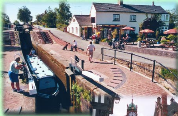
◀ Grindley Brook staircase on the Llangollen canal.
